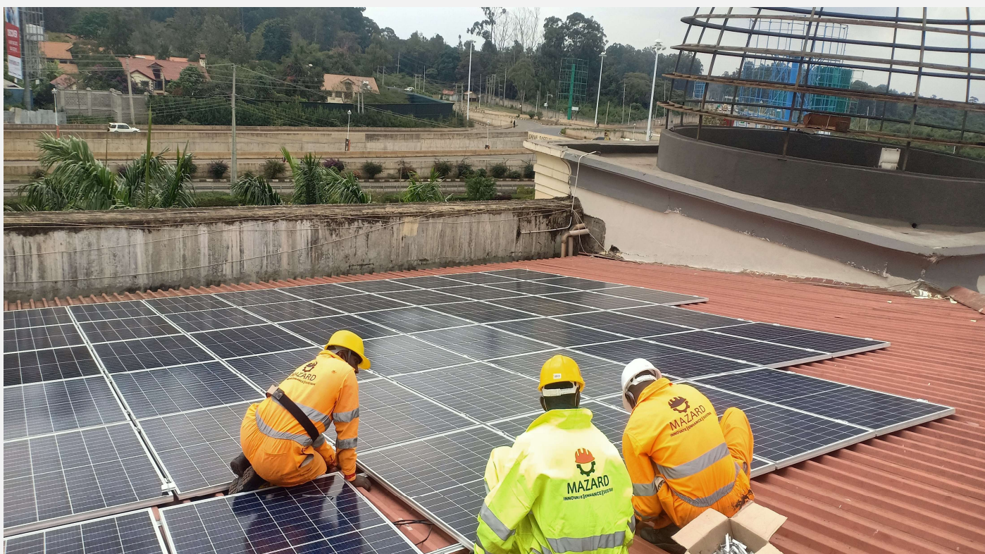
Galleria Mall Roof
